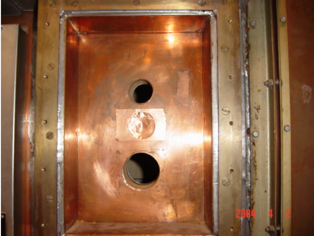
Figure - 7: Room 11M (Test Room) Outer Mounting Plate (View from outside chamber)
