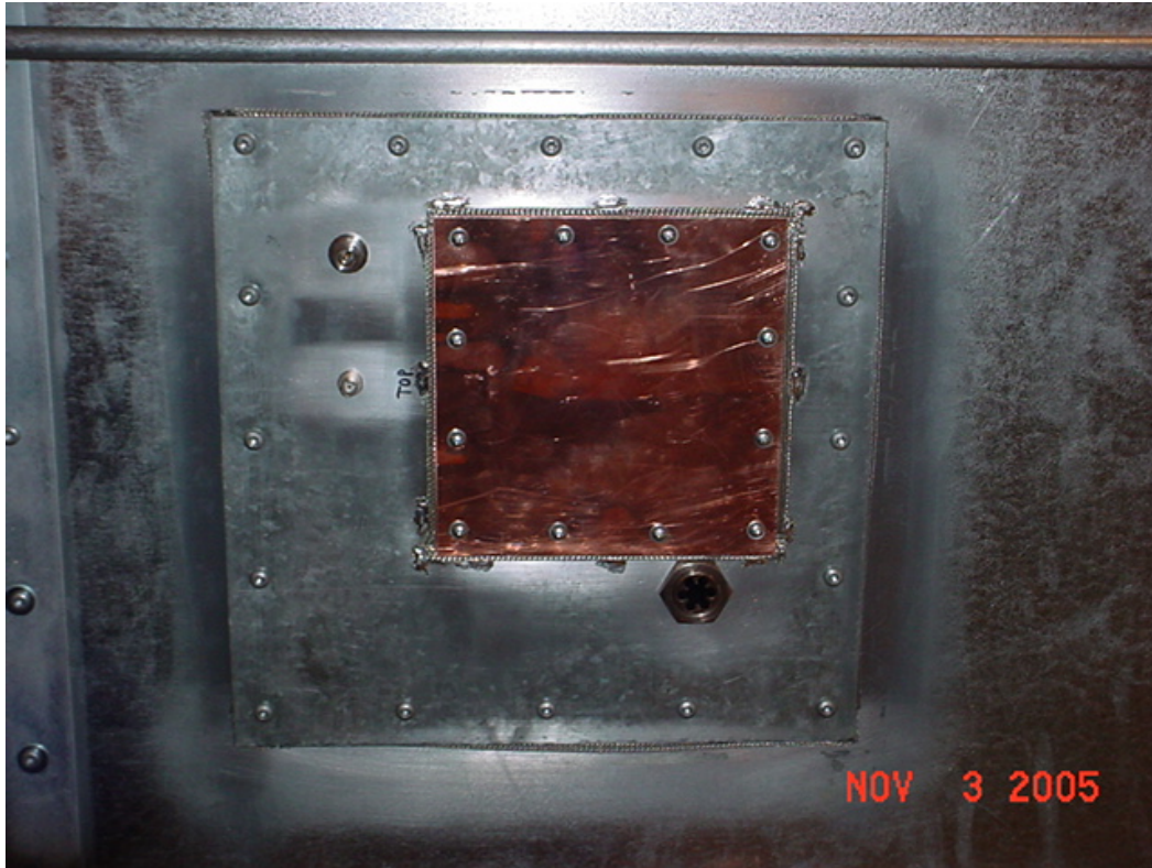
Room 24S (Test Room) Inner Mounting Plate Plate #1
