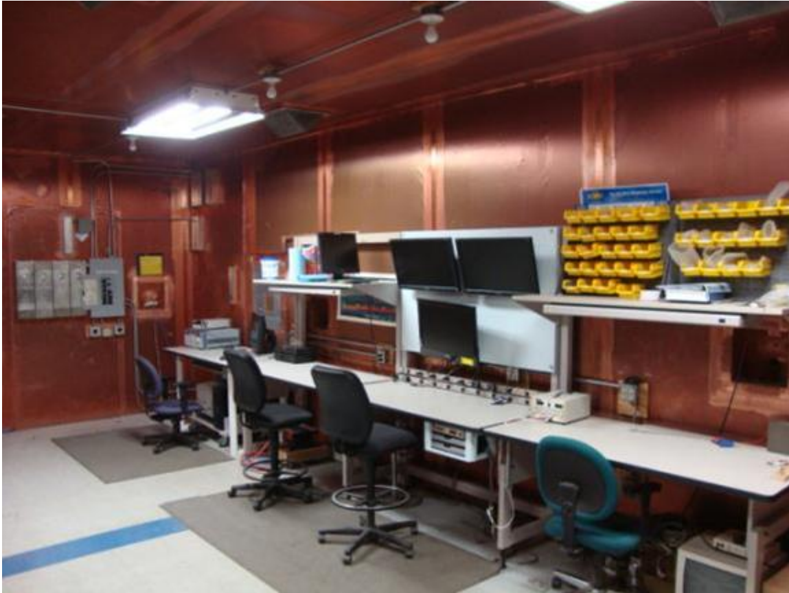
Figure – 3: Room 22P (Monitor Room)
