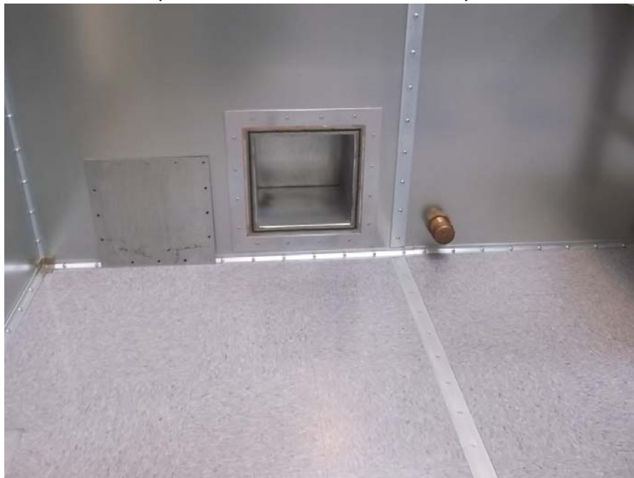
Figure – 4: Room R11P (Monitor Room) Lower Waveguide opening (View from inside chamber)
