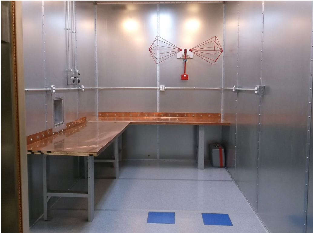
Figure - 2: Room 11P (Monitor Room)
