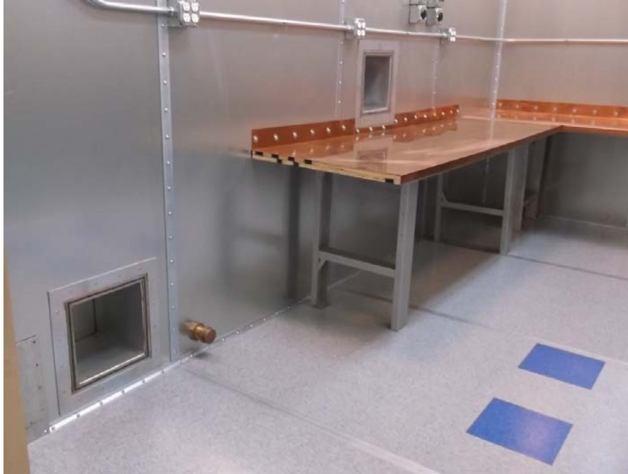
Figure – 3: Room R11P (Monitor Room) Upper & Lower waveguide locations (View from outside chamber)
