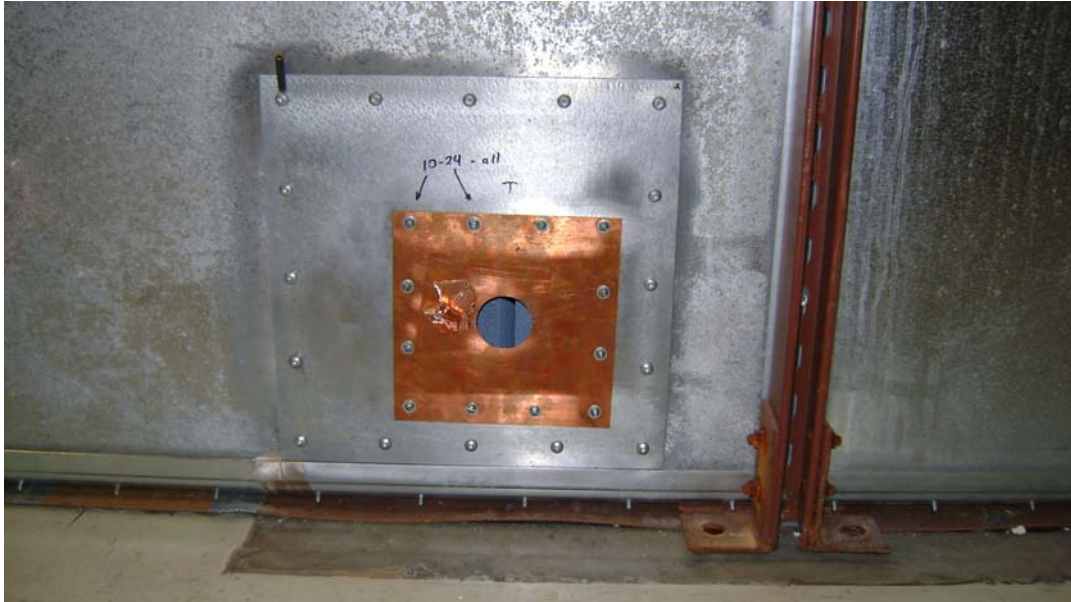
Figure – 6: Monitor room plate #1
