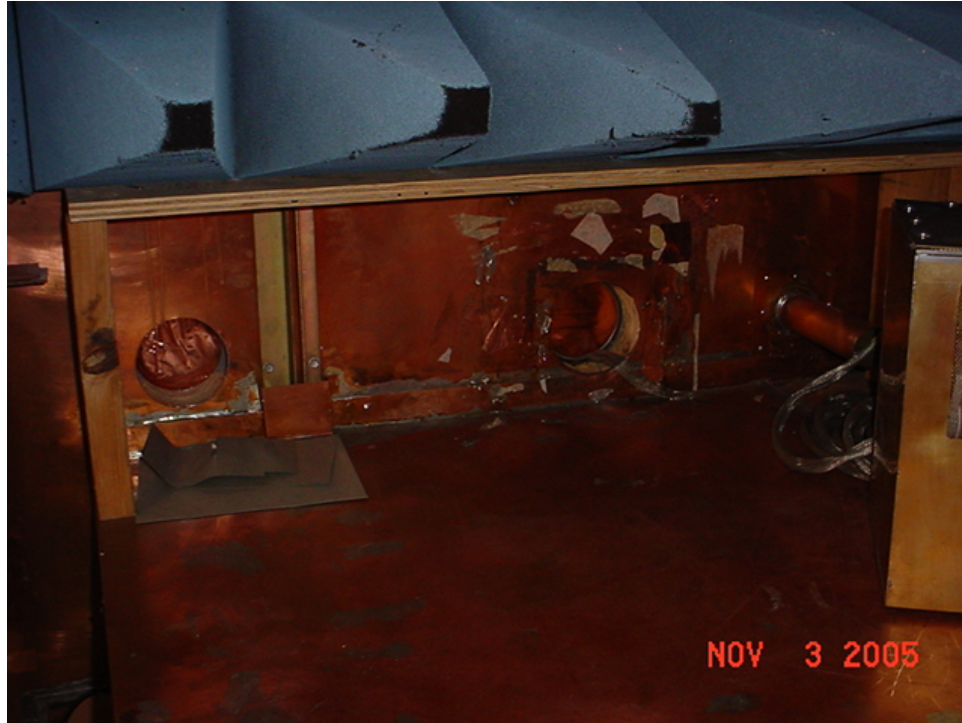
Figure - 4: Room 19M Common Wall Openings
