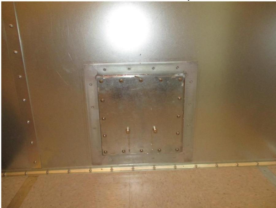
**Figure – 4: Room R12P (Monitor Room) Lower Waveguide opening (View from inside chamber)**
