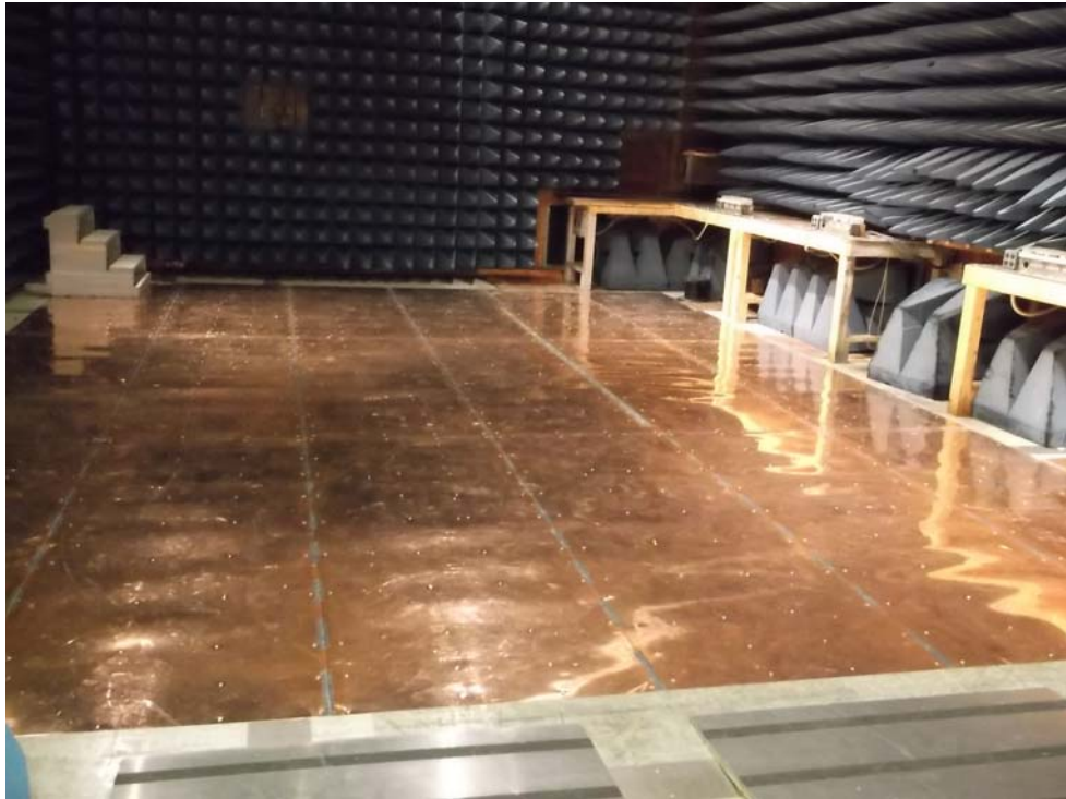
Figure – 1a: Room 23M
