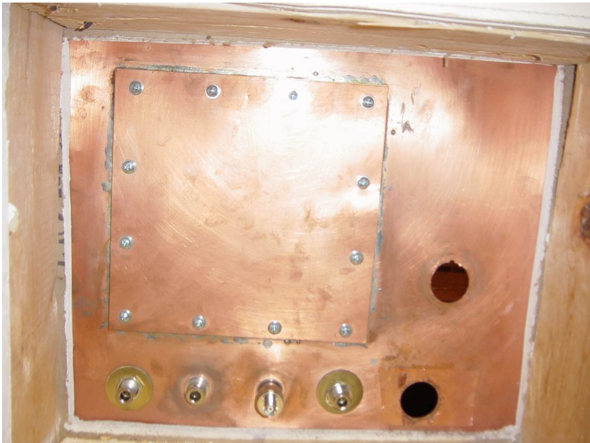
Figure – 6: Equipment Interface Mounting Plate #2 w/ Universal plate See Universal Plate Figure 7 for Inner Plate Dimensions
