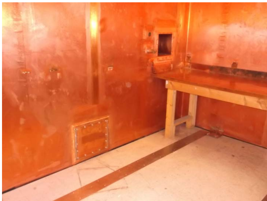
Figure – 9: Room 23M panel below ground plane to 23L under the ground plane. 13 ¾ inch by 11 ½ inch high opening (Plate #3)
