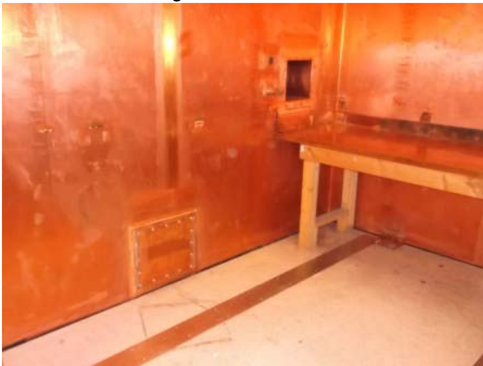
Figure – 2b: Room 23L
